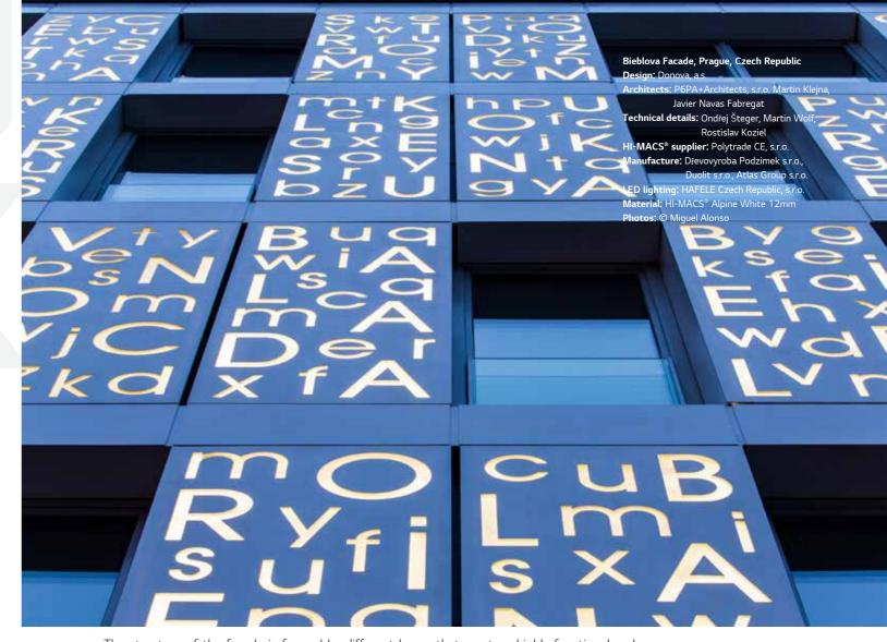
The structure of the facade is formed by different layers that create a highly functional and extremely aesthetic cladding element. The external covering comprises a 12-mm layer of HI-MACS®, a layer of 8-mm transparent acrylic glass, and a third layer of black acrylic glass underneath. The hidden load-bearing element of the facade is a steel structure.
